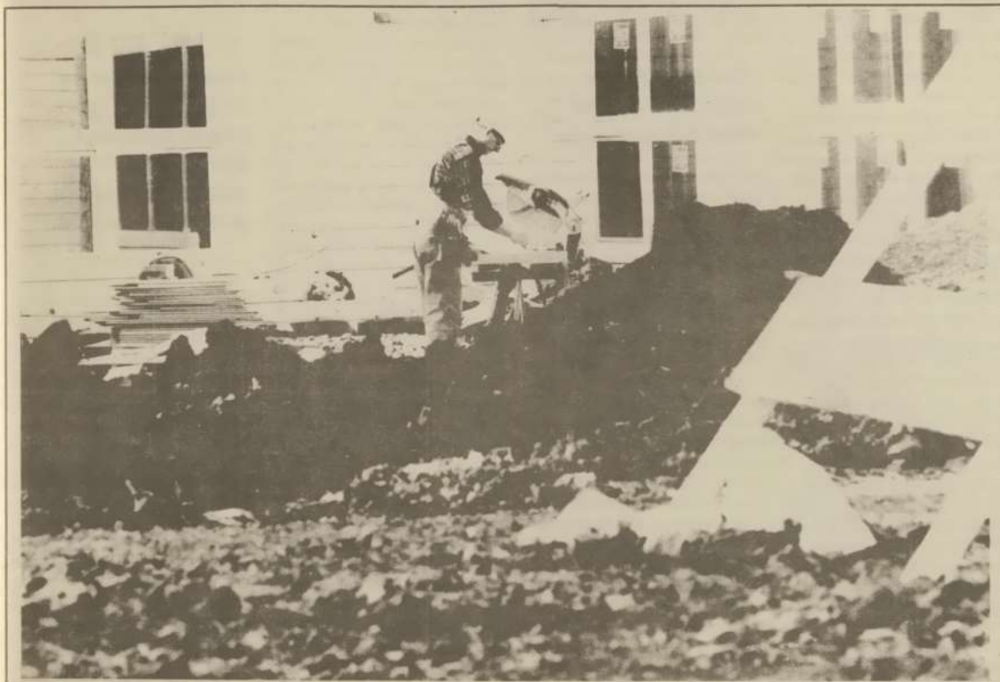
Construction continues on the new CCC Day Care Center. Workers plan to finish by spring term. Several other buildings are also under construction and they are all progressing well.
