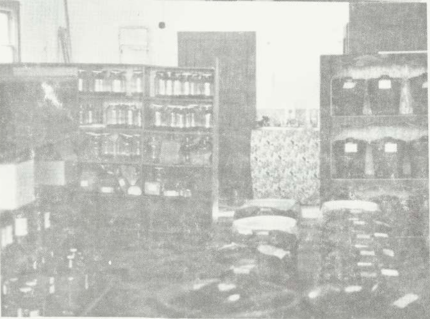
Volunteer carpenter puts finishing touches on remodeling of new Oregon City food co-op. Below, the 'finished product' opened recently for business in all types of bulk food.
