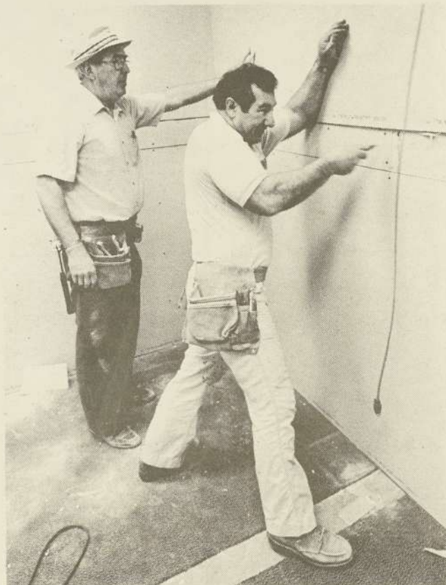
Bus Morrow (left) and Jerry Kadlec of Howard Brewton General Contractors put sheetrock into Kevin McMurdo's new office.
