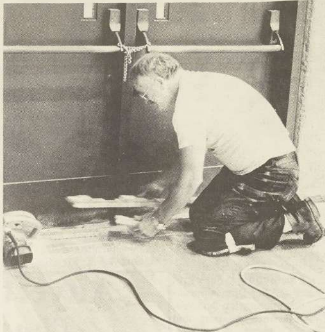
STEVE BIGELOW OF Ryerson Hardwood Floors in Portland lays custom cut wood for threshold
