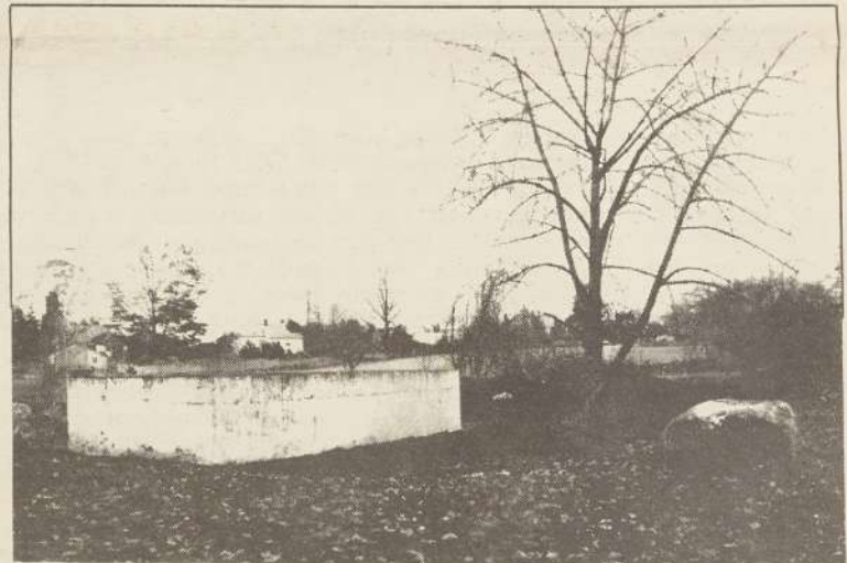
THEN AND NOW--ELC site (above) Below is completed tank that will be dedicated and christened May 11.
