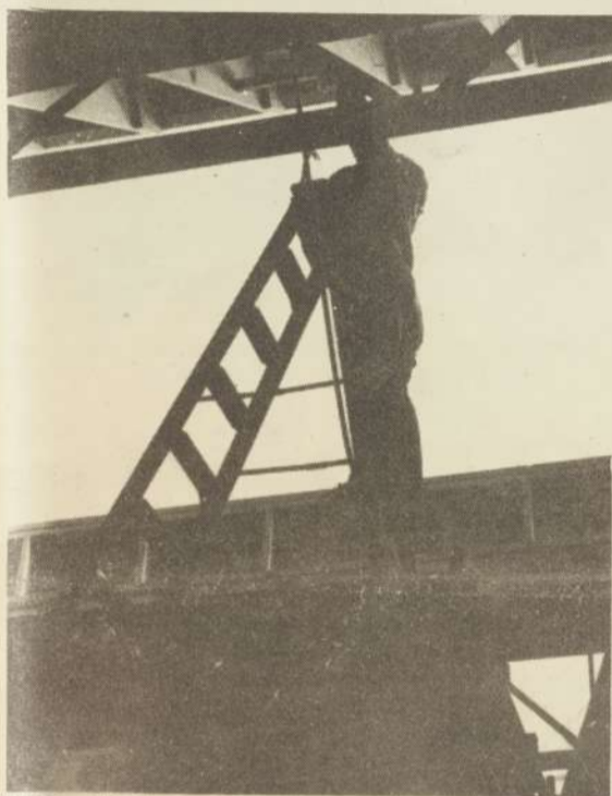
POUND —Worker tends to new science facility. Photo by Ramona Isackson.
