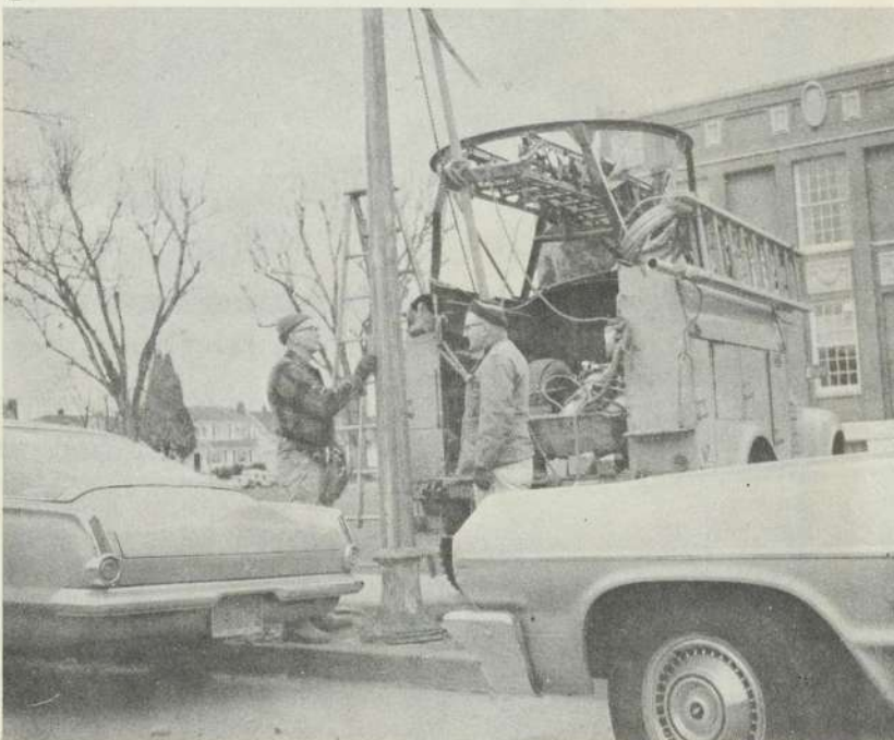
'Welp, what color?' During the last week members of the electric company have been painting and repairing the lights that surround the campus. Work began on the lights earlier this year and should be completed in the near future.
