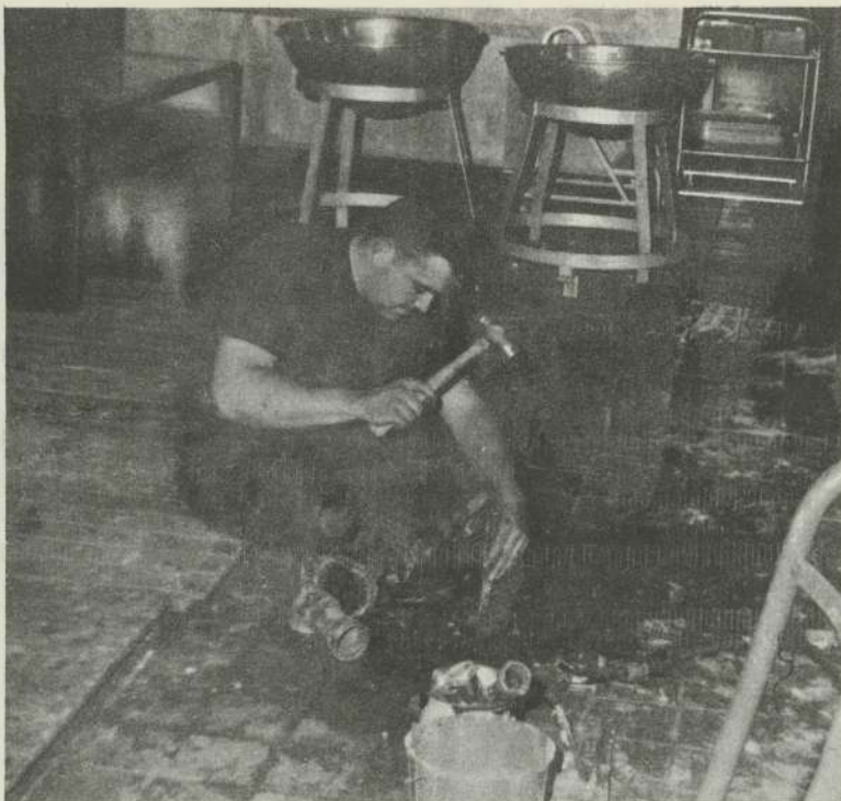
Kitchen improvement Jerry Krause, assistant head plumber from the school district Maintenance department, installs new floor drain especially designed for kitchen improvement in the space formerly occupied by a dishwasher which was relocated.
