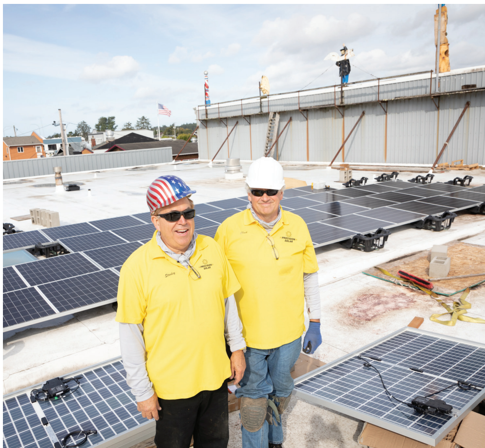
Stan Tussing and Chuck Waddell of Precision Solar, Heating & Indoor Air Quality stand next to a 20,000-watt solar panel installation atop Marsh's Free Museum in Long Beach.
