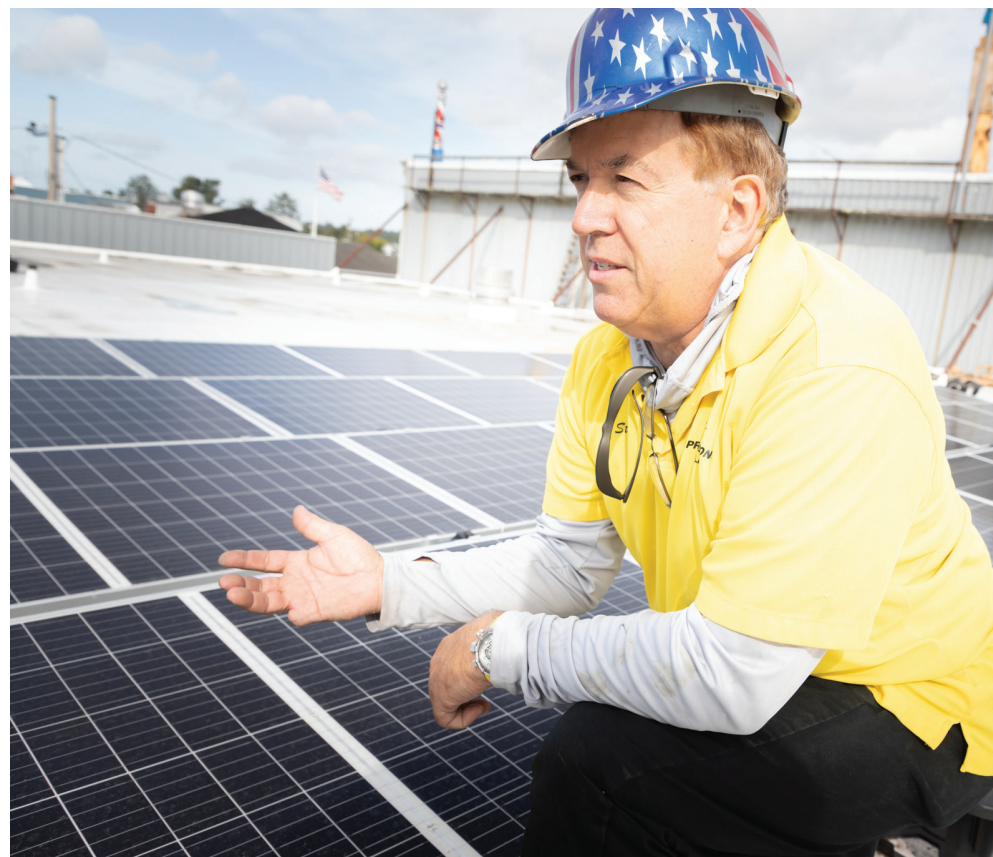
Precision Solar, Heating & Indoor Air Quality owner Stan Tussing observes the work completed at Marsh's Free Museum, a 100-year-old Long Beach business.
