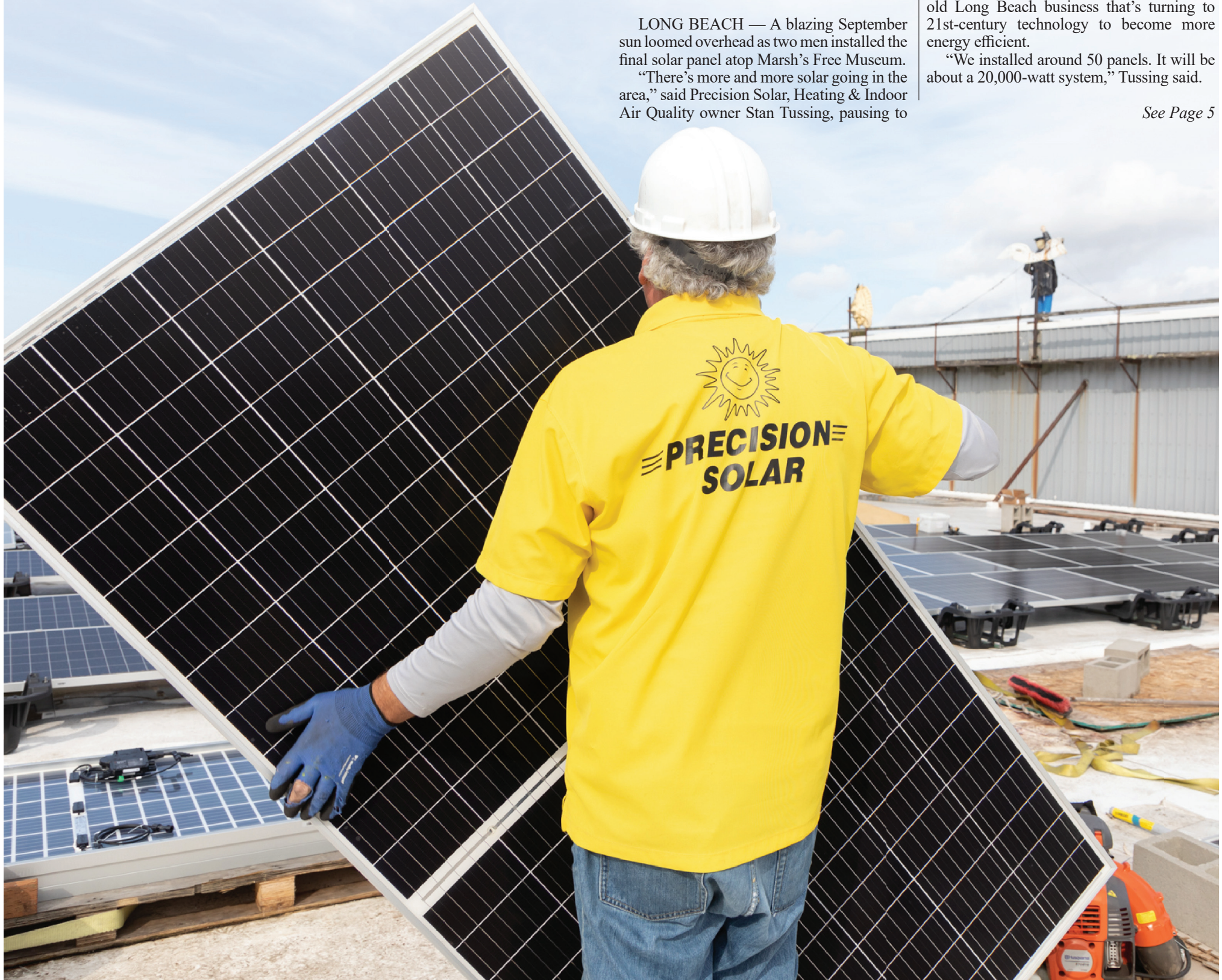
Chuck Waddell installs solar panels at Marsh's Free Museum in Long Beach.
