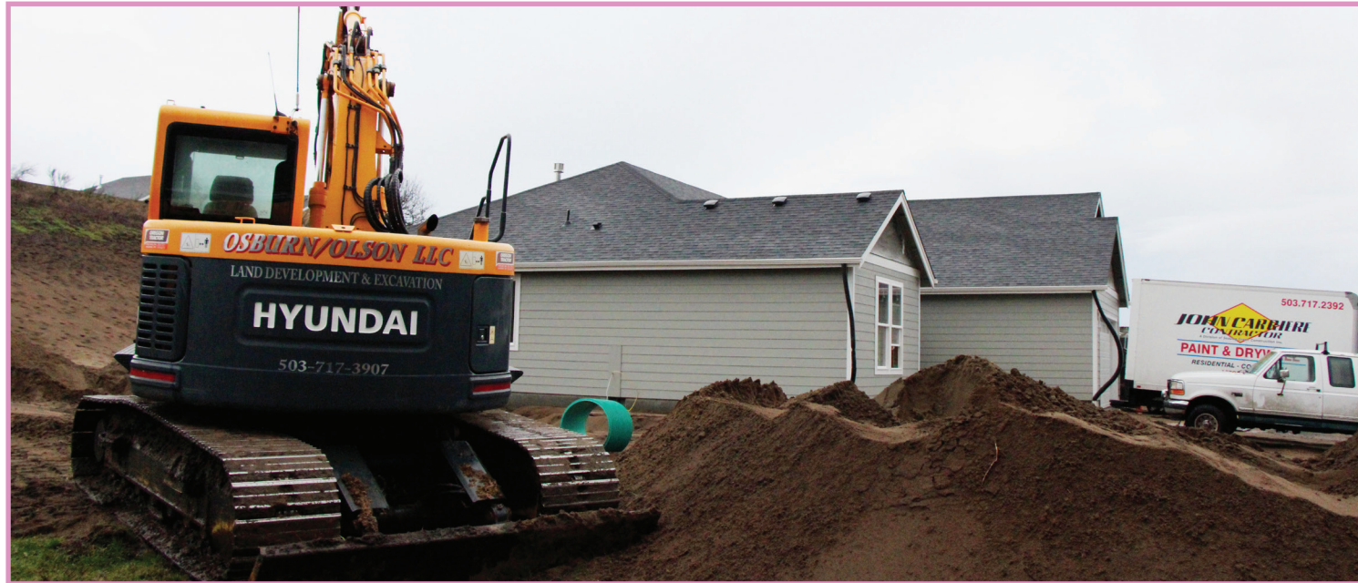
Housing development is underway between Warrenton and Gearhart.
