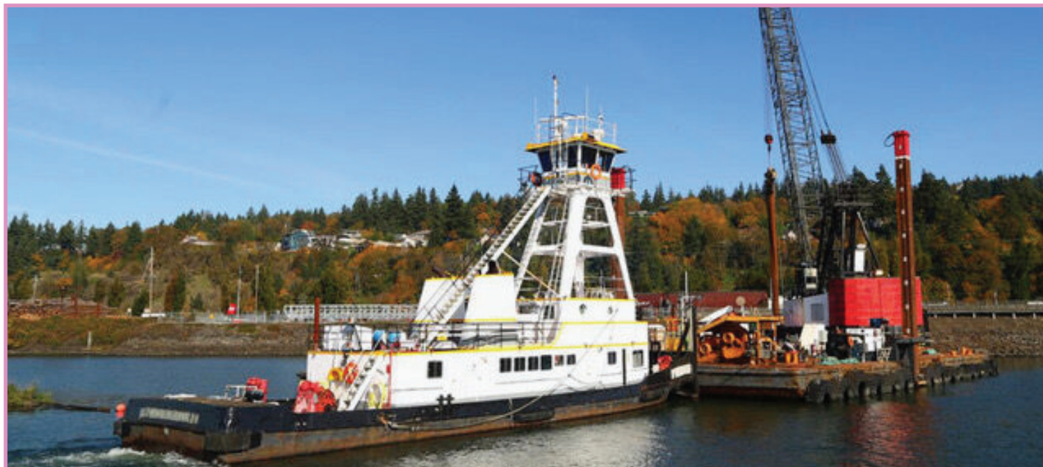
The Voyager pushes the DB Beaver crane at the Port of Kalama in 2019.
