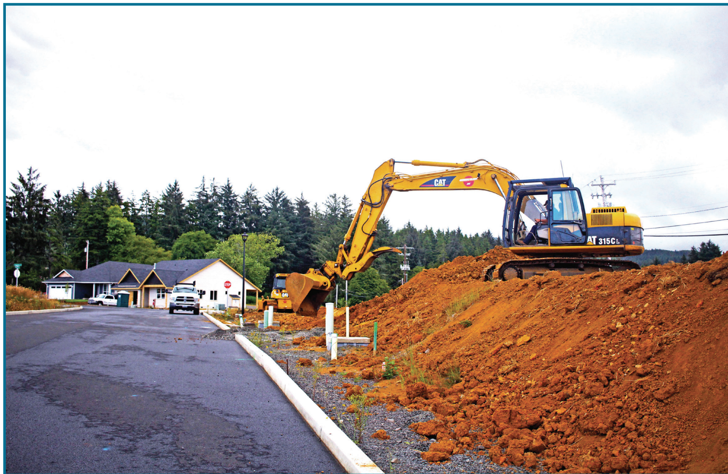
Contractors work on the Blue Heron Pointe subdivision in Seaside.
