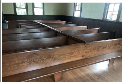
Oysterville Church WA - Pew Restoration
