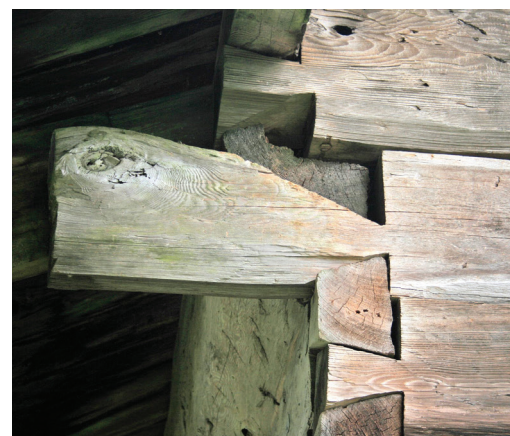
Lindgren added an artistic touch, extending the dovetail joint near the eaves.
