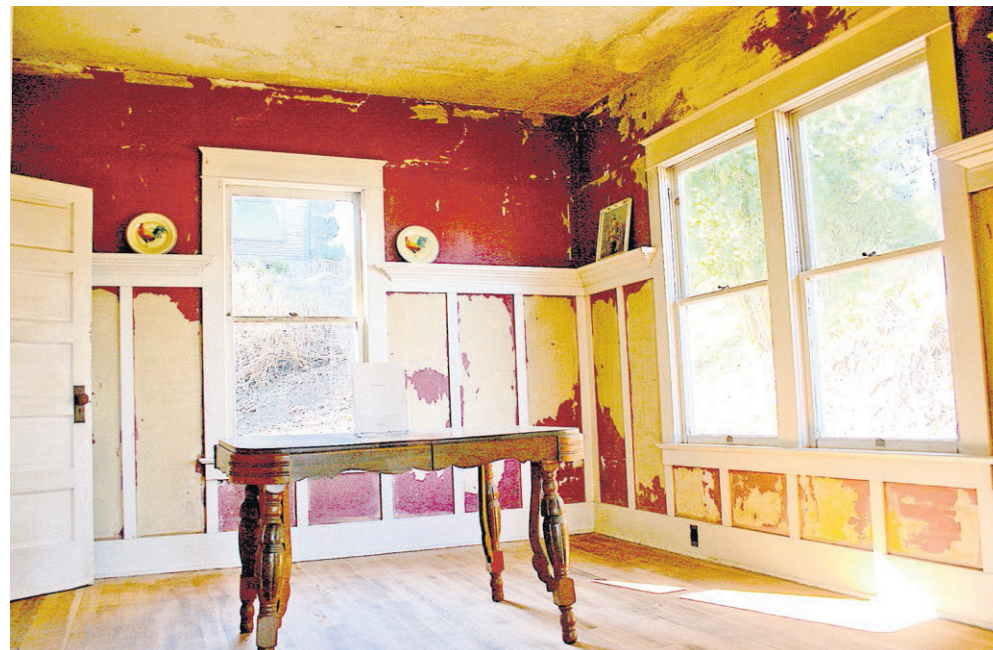
The dining room is wrapped in wainscoting.
