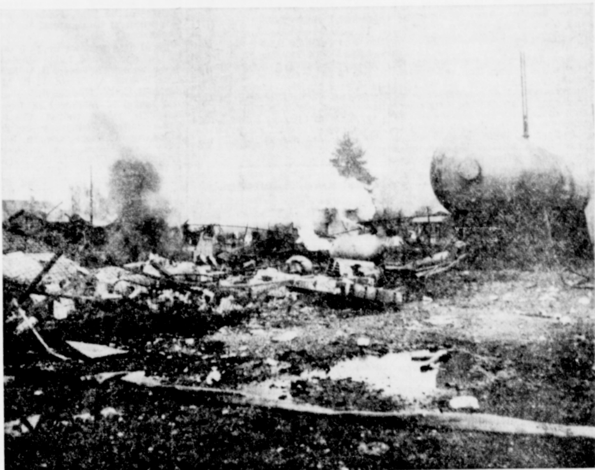
TAKEN FROM ANOTHER ANGLE than pictures of the Cottage Grove Gas company fire published last week is this one which shows the mass of twisted wreckage. In the middle is a 1000-gallon tank such as is delivered to larger commercial users in rural areas. It was knocked over in the explosion and its valve knocked off. Gas escaping from the valve burst into flame and burned for several hours.
