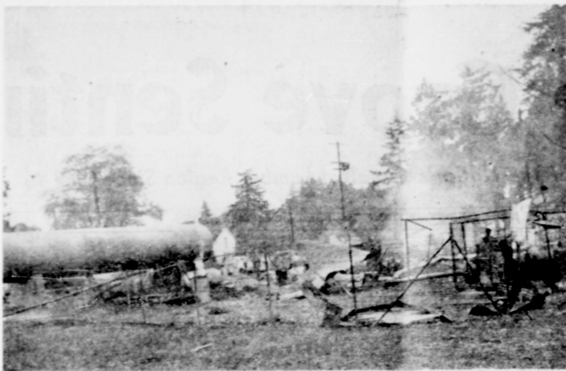
AMAZINGLY, THE PROPANE TANK, shown here, was not damaged although it was just alongside the one which did explode and another smaller one which was opened and which can be seen here burning.
