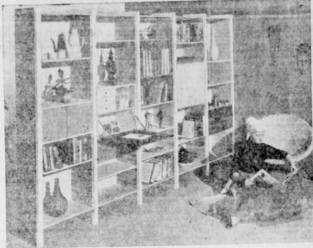
The unit storage wall is the name for this beautiful interior stud-partition treatment. Most interior stud-partitions occupy valuable space, but this storage wall has been designed to utilize that space into many attractive and usable storage spaces. Texture One-Eleven (grooved plywood) has been adapted to support shelves so that they can slide into grooves at varying and usually adjustable heights.
