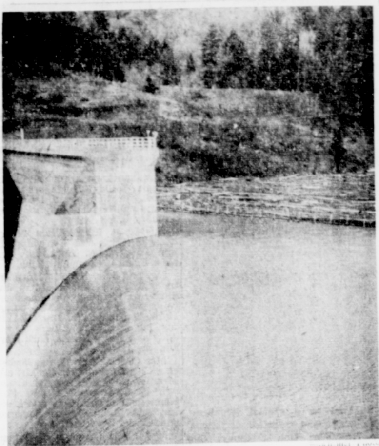
AT A CREST OF 3.2 FEET over the spillway, Dorena Dam releases some of the "would-be" flood waters that had stored up. The crest was reached Friday, December 23.
