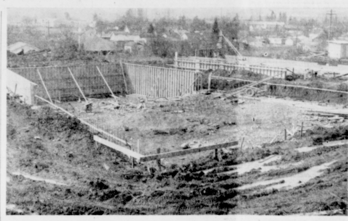
CEMENT FORMS FOR GROVE'S NEW SWIMMING POOL and bathhouse were almost completed as of late last week. Work on the pool is progressing at the expected rate, and it should be ready for use by Centennial week.
