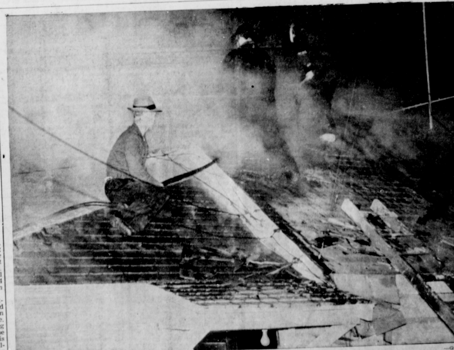
A GROUP OF COTTAGE GROVE'S VOLUNTEER FIREMEN (left to right) Albert Stacks, Jim Pynch and Jim Shirley, are shown extinguishing flames on the roof of the Melvin Tonole residence, which was badly damaged by fire. Flames, according to Tonole, broke out at 4:50 Tuesday morning. The interior of the living room was gutted and the remaining four rooms badly damaged by smoke.
