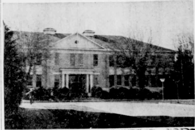
THIS STRAIGHT ON VIEW is Jefferson School one year BC (Before Chopping) trees. The three trees in front of the school were not only blotting out the light from the classrooms, but made it impossible to grow a lawn underneath, their rotten limbs were a hazard and had to be constantly topped. The trees were taken out, leaving the picture below.
