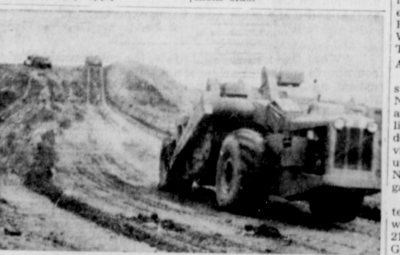
A MONSTROUS "TURNAPULL" roars down the mountainside in back of the high school with 15 yards of dirt. Construction on the new highway in this section has been going on for three weeks.
