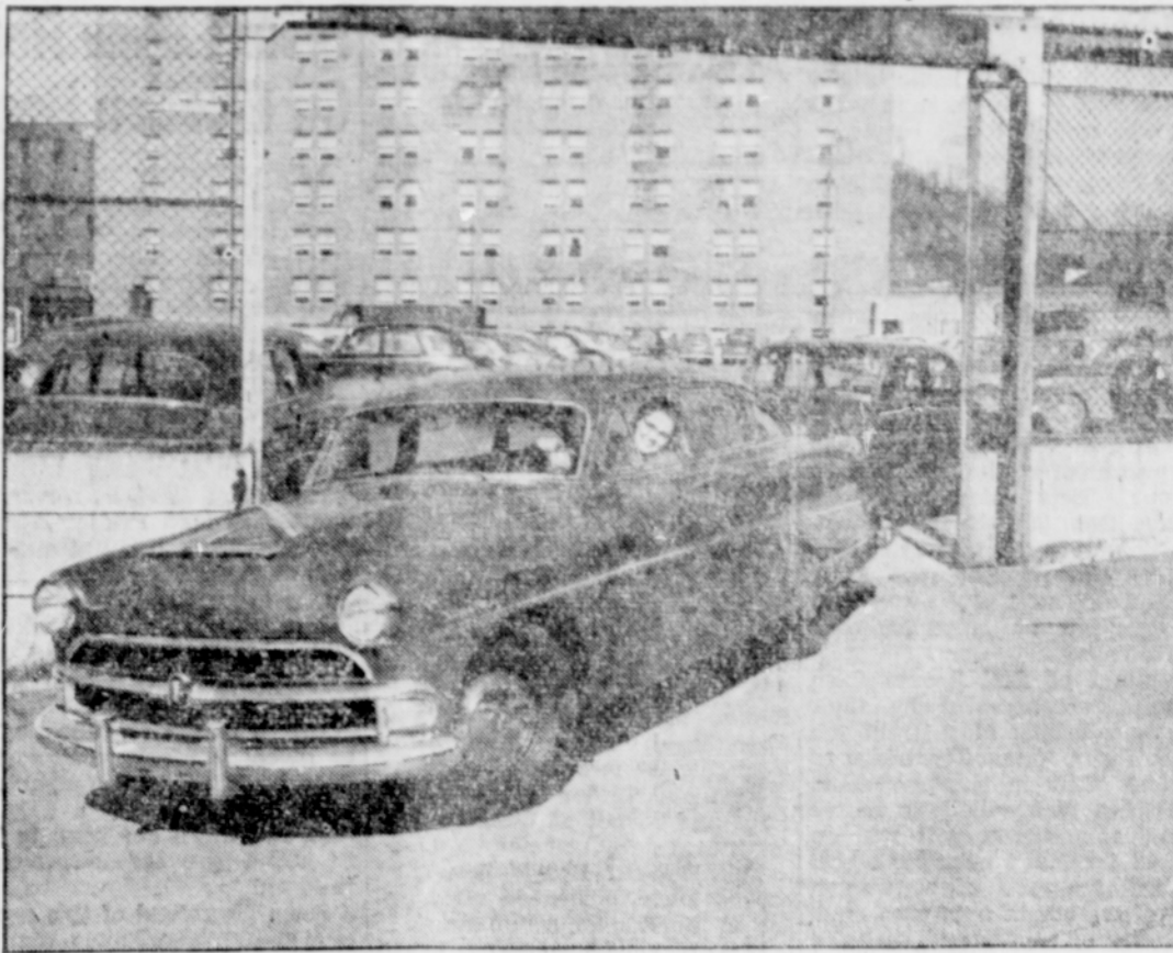
BLUEFIELD, WEST VIRGINIA, SHOPPERS can drive directly from the roof of the parking garage to an adjacent street. The garage was planned to suit the hilly streets of the city.
