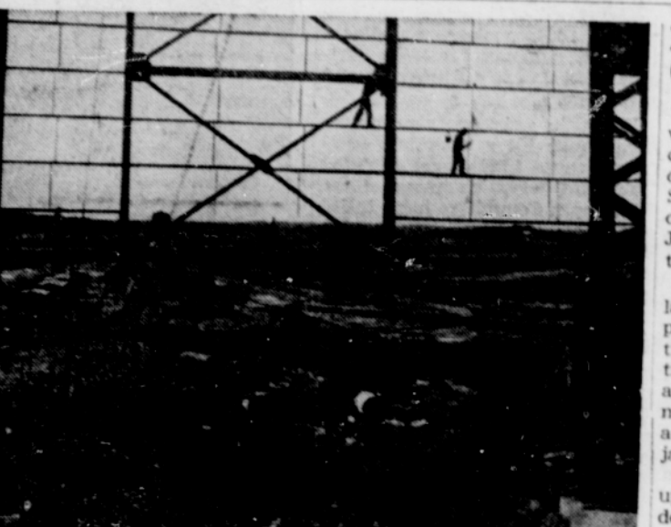
NEW STEEL FACILITIES TAKE SHAPE —Workman painting braces on the end of a new open hearth building. This new plant is part of the National Production Authority's program for the expansion of basic industry. It will play a major part in raising our steel capacity to 120 million ingot tons by the beginning of 1954.
