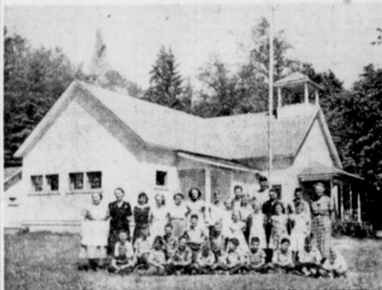
Blue Mt. school as it looks today with its clean coat of white. Not seen in picture are lunchroom and gym. Entrance part of school looks like old one-room schoolhouse, might have been part of original building. A total of 28 students pose with their teachers and cook. Mrs. Berta McGuire, (standing, far left) cook; Mona Moore, next to Mrs. McGuire, upper grades teacher, and Mrs. Louise Wickendoll (far right, standing) principal and lower grade teacher.
