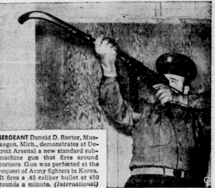
SERGEANT Donald D. Rector, Muskegon, Mich., demonstrates at Detroit Arsenal a new standard sub-machine gun that fires around corners. Gun was perfected at the request of Army fighters in Korea. It fires a .45 caliber bullet at 450 rounds a minute. (International)
