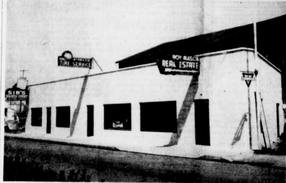
The new Bartels building, occupied by Roy Mason Real Estate, Sib's Radiator Shop, and McKenzie Tire Service, was built by P. J. Bush and Sons, Contractors. The firms opened for business two weeks ago. (Sentinel Photo)
