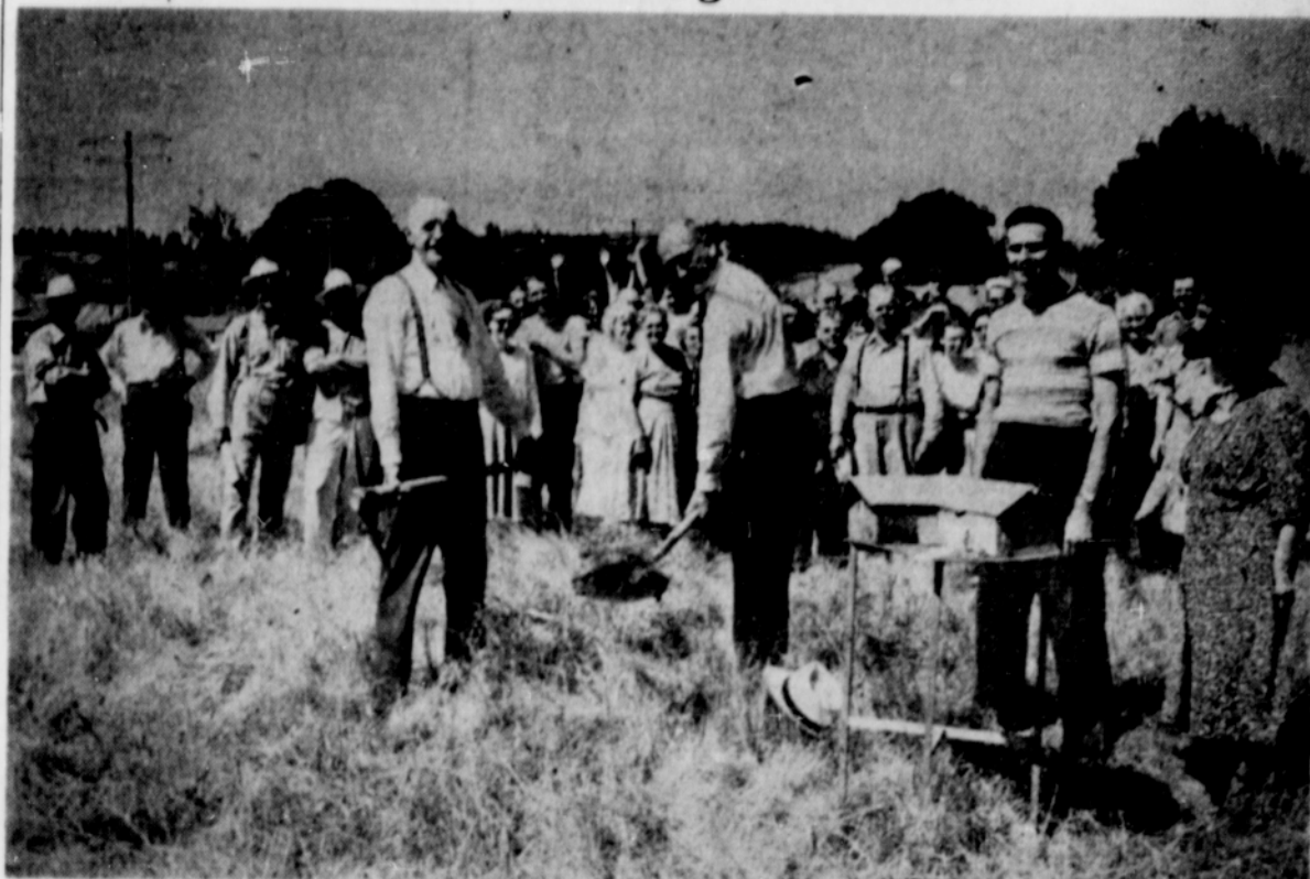
Elder Lloyd E. Briggs, president of the Oregon Conference of Seventh-day Adventists, turns the first shovel-full at the groundbreaking ceremony of the new S.D.A. church Aug. 20. Also participating in the program were Mayor Frank Doleman, Elder Walter Blehm, and Mrs. Gertrude Trask. In the foreground is a model of the new church.
