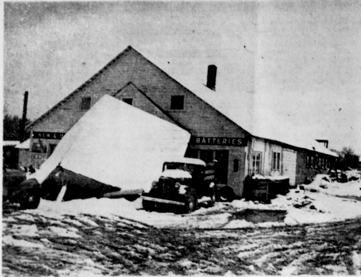
Among the victims of the early snowfall was the M. & S. Auto Service on north 99 highway which lost its marquee, when heavy snow caved in the front.
