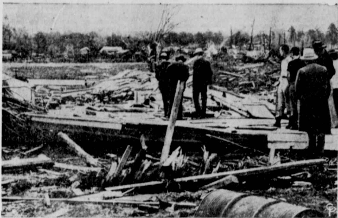
CURIOUS SPECTATORS view the splintered wreckage of houses that were in the path of the tornado which smashed Whelen Springs, Ark. In foreground is all that remained of the home of Mrs. James H. Van Meter, 60, who was killed when the twister chopped its way through the town. Tornado winds which hopped across five southern states left at least twenty-eight persons dead and scores injured. (International Soundphoto)
