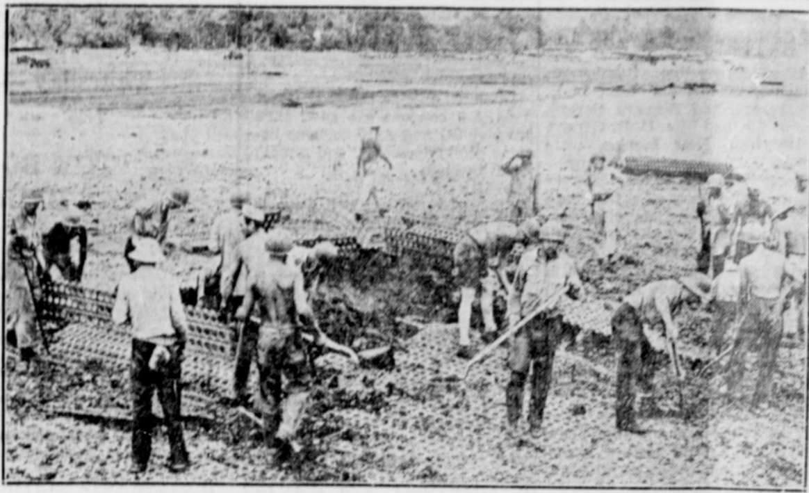
LIGHTNING REPAIRS OF BOMB DAMAGE —Sometimes it is merely a matter of minutes after enemy aircraft bomb an airfield until U. S. Army Aviation Engineers are on the job repairing the damage. The portable steel landing mat is replaced and the runways are available for American planes in the shortest possible time. This scene at Guadalcanal is typical of the efficient work in restoring a shattered airfield. The Seabees, naval counterpart of the Aviation Engineers, have made splendid records in this theater of operations.
