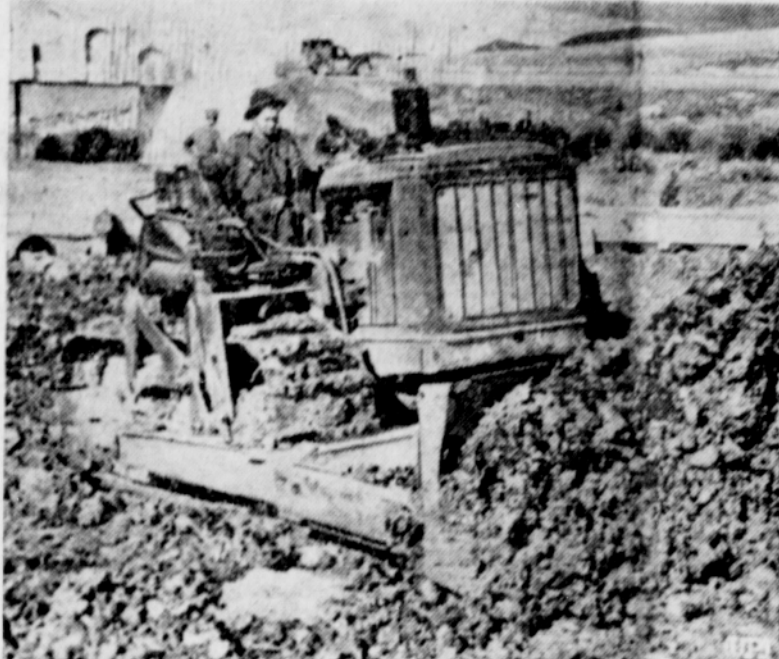
Mud is only one of the obstacles which confront the Allies in North Africa. Making bad roads passable for jeeps and tanks and troops is a big job. Here is an American construction gang attacking the problem.
