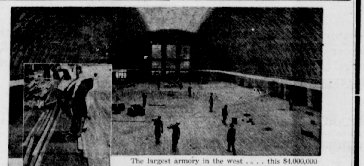
The largest armory in the west . . . this $4,000,000 building has 32,000 square feet of wood flooring and timber Lamella roof!
