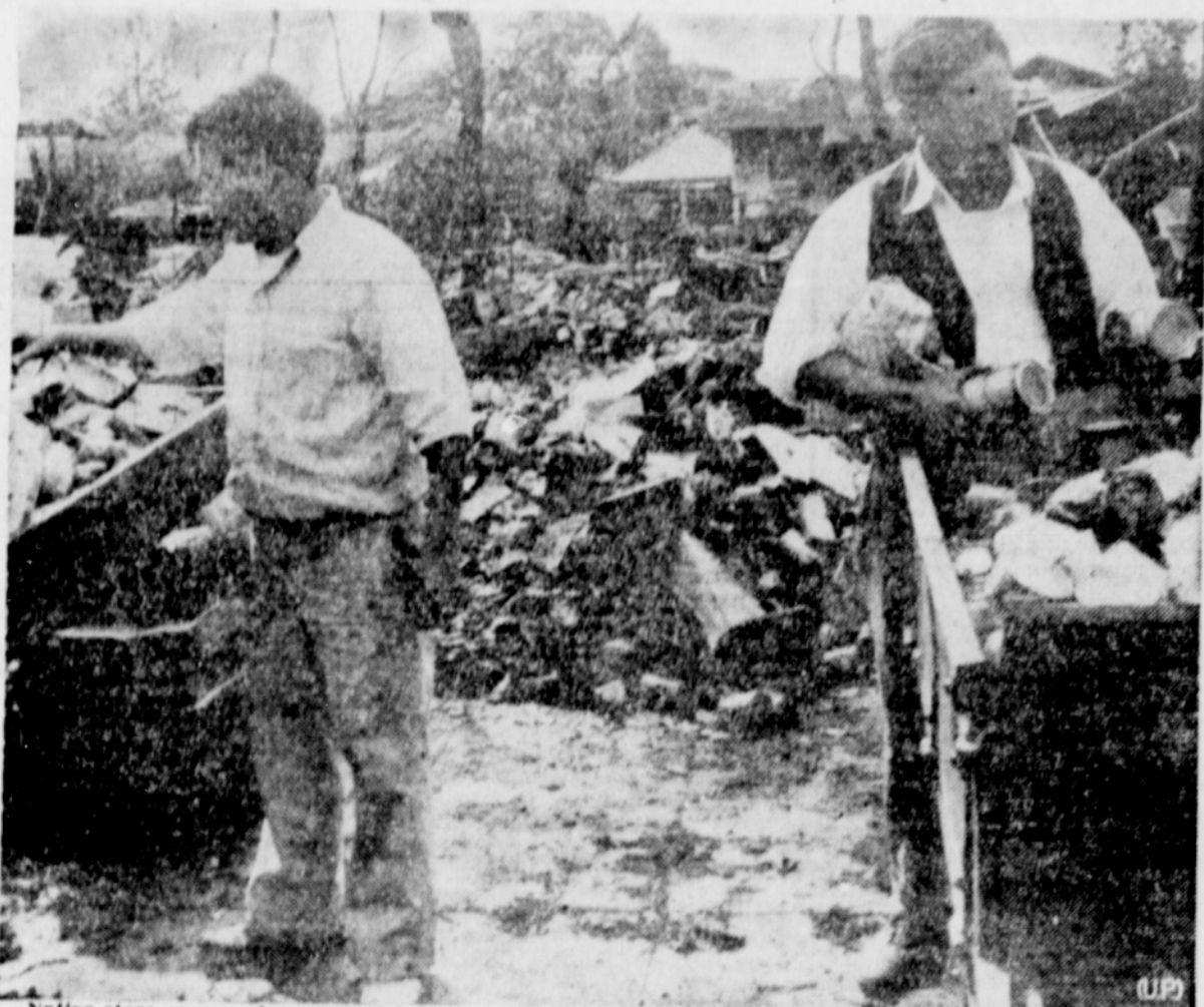
Native store owners clear away debris caused by Jap bombs and salvage what's left of value in a whole block of small establishments wiped out by fire and explosions in Honolulu in Dec. 7 attack. (Photo passed by U. S. Censor.)
