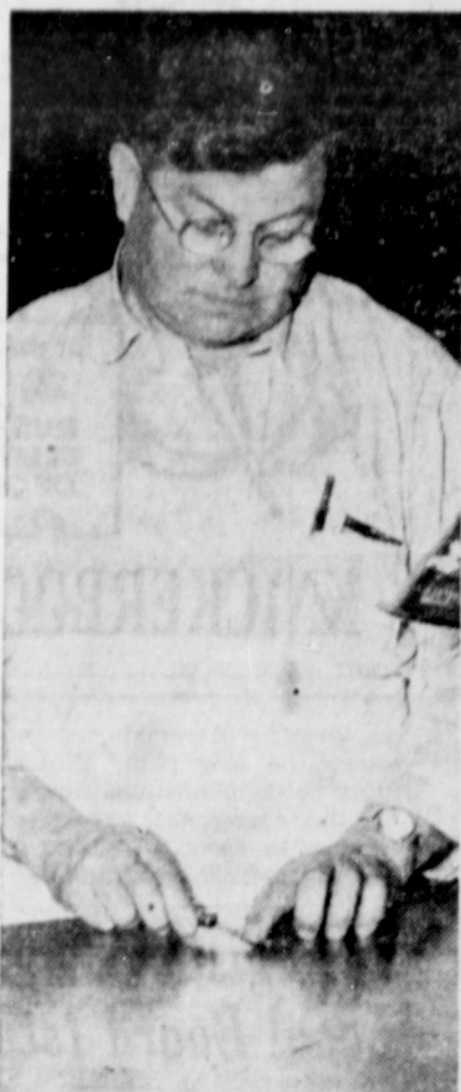
Thinner than a frog's hair or gnat's eyebrow are shavings removed by this highly skilled workman from 900-pound "thrust shoe" that must carry 900-ton rotating parts of 108,000-kilowatt generator at Grand Coulee Dam, Washington. It will produce current in August, 1941. Shoe's surface must be so accurate that microscopic oil film will not "break" at "high" spots by tremendous weight of moving parts shown.
