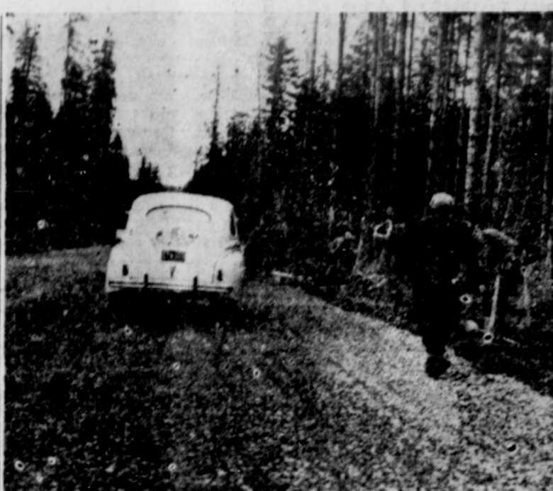
The motorloggers stopped on a graded section of the highway to "kibitz" WPA workers leveling the crushed surfacing rock.
