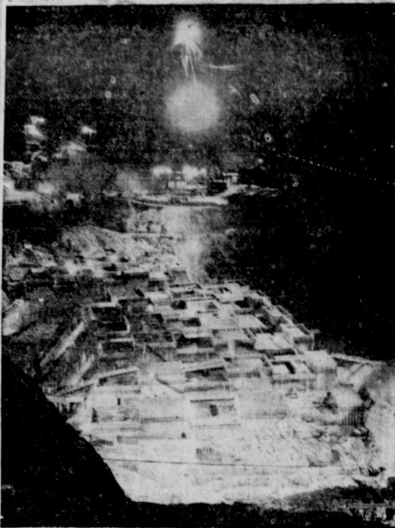
Powerful floodlights, permitting 24-hour work schedules, illuminate giant Shasta Dam project in this dramatic photograph. This view of world's second largest concrete dam taken from top of east abutment.
