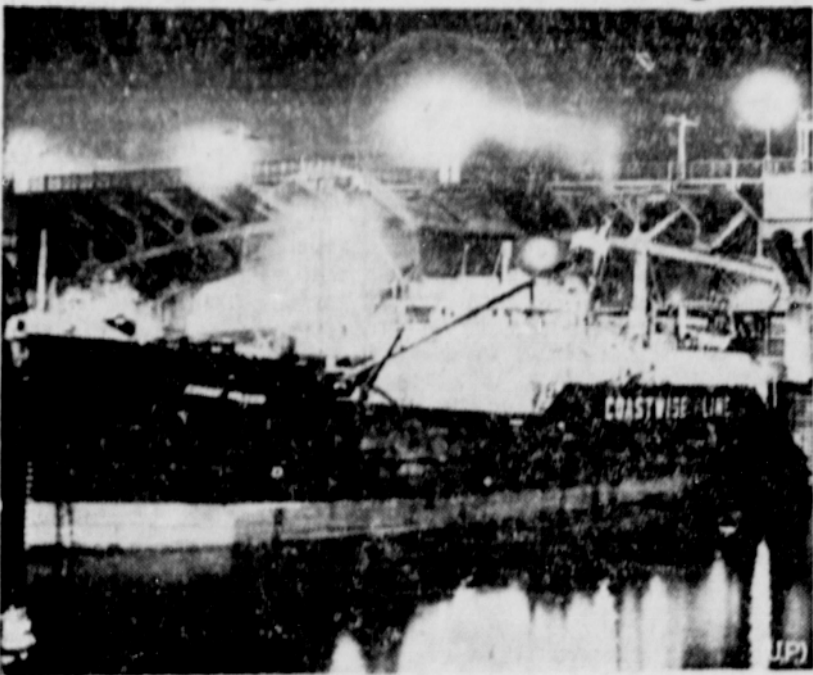
This is what happens when a ship is smacked by a drawbridge. Freighter Coast Miller was under Burnside Drawbridge at Portland, Ore., when mechanism failed. Span crashed on ship. Note how ship's funnel is bent back. Damage was considerable but there were no casualties.
