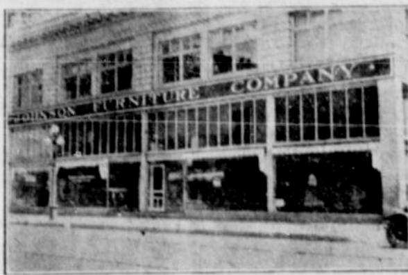
Front View of the Johnson Furniture Company.
