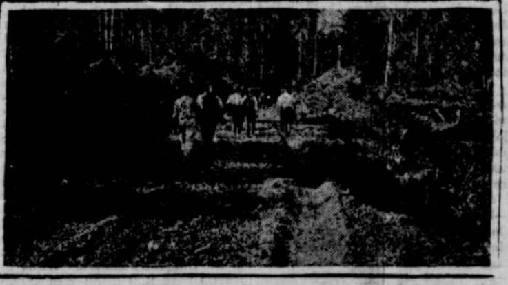
Upper Left—Cottage Grove Business Men Board Train. Upper Right—Huge Steam Shovel at Work. Center—New Bridge, 795 Feet Long. Lower—Scene Along Grade.
