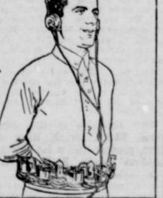
ideal for the hiker. It is a three-tube receiver, operating on small batteries and is complete in all details. The instruments are fastened to a canvas web belt, and each tube has its own rheostat; a potentiometer is also provided. The set has sufficient power to operate a loud speaker, and it is said that stations as far away as Chicago have been heard on it. The antenna consists of fine wire sewn between two canvas sheets so that it may be carried under the shirt, or in a pocket.
