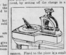
touchhole of the gun in such a way that they do not reach the powder until the sun's position is directly in line with a tiny opening. The supports of the "alarm" are arranged to adjust it to the light beams at the same time every day of the year. Often the device fails to work because
