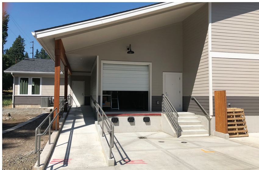
Vernonia Cares now has their own loading dock. At the old location freight was delivered to the sidewalk in front of the building and then moved by hand truck up a ramp and into the warehouse.
