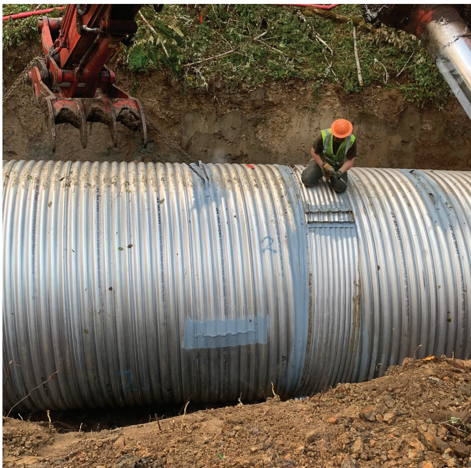
Above & right: West Coast Road Construction removed a culvert on Kauppi Lake Crossing and replaced it with this 11 foot fish passable culvert.
