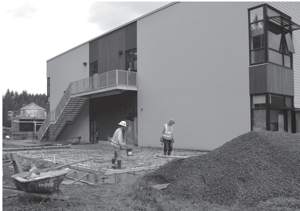
Construction progress on the art room addition on May 15, 2020.
