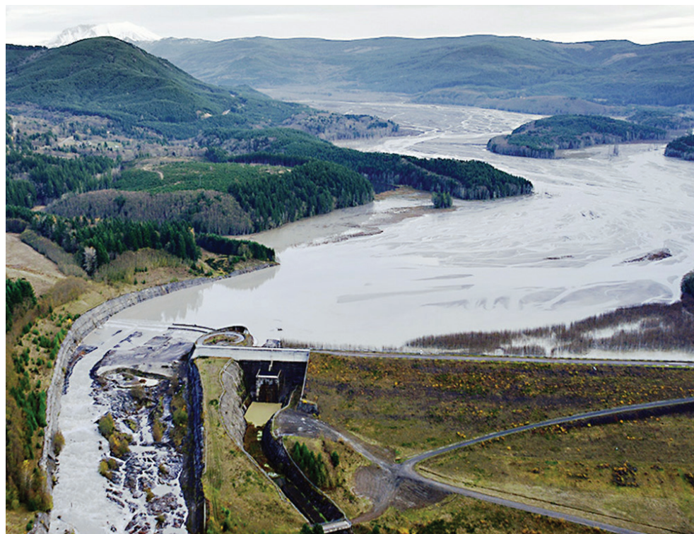
The sediment retention structure and upstream sediment plain on the North Fork Toutle River, flowing out of Spirit Lake. Photo Credit: U.S. Army Corps of Engineers
