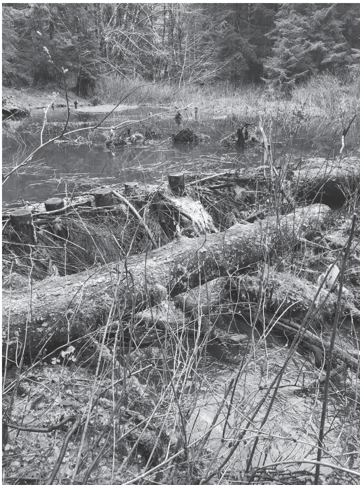
BDAs are constructed by pounding in a row of vertical Douglas fir posts across a stream, which are then interwoven with vine maple or Doug fir limbs. Ideally the BDA will provide a prime location for beavers to naturally colonize.
