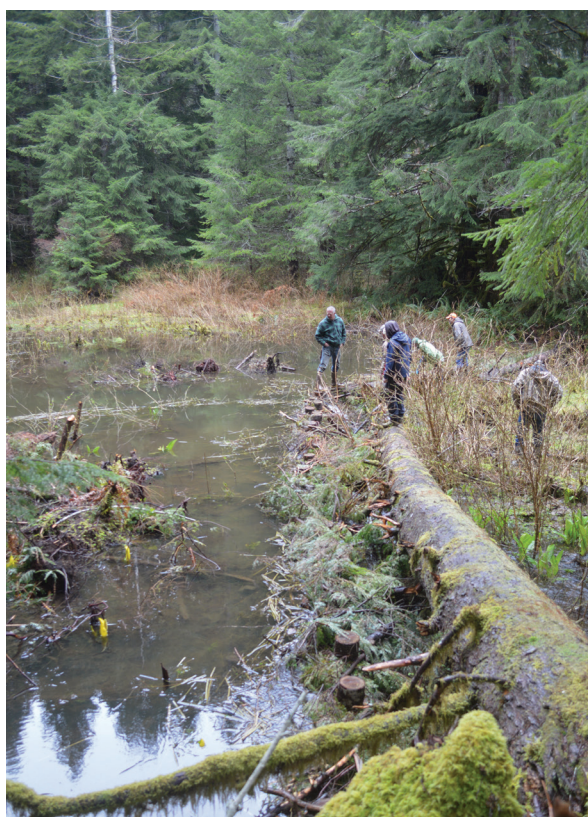
A Beaver Dam Analogue (BDA) constructed in the Tillamook State Forest, part of a pilot project being managed by Upper Nehalem Watershed Council.
